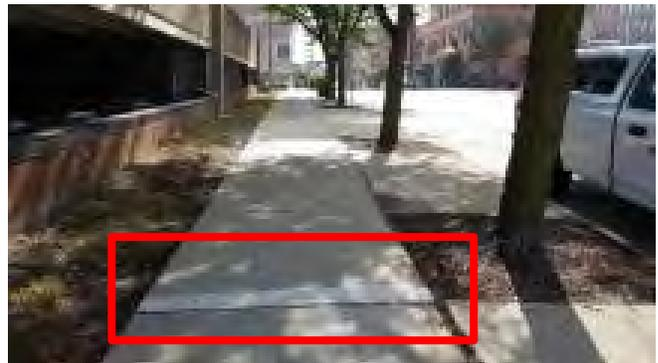
**Unit of measurement:** The City measures grinding in inch-feet by taking the highest part of the grind plus the lowest part of the grind, dividing by two, and multiplying this average grind height by the length of the grind. Height is measured to the nearest 1/8th inch.
