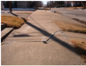
Figure 19: Fair + (5) - Might be a hindrance to some pedestrians, but functionality acceptable to most.
