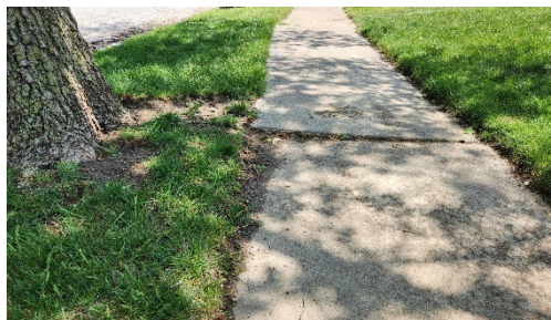
Figure 31: Example of tree heaving
