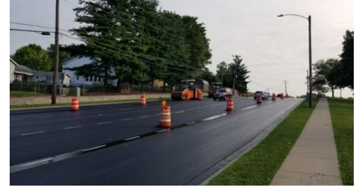
Figure 39: Rolling after resurfacing
