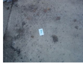
Figure 17: Good + (7) - Weathering and minor defects are becoming visible. Still functional.
