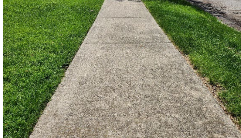
Figure 25: Old sidewalk but still good
