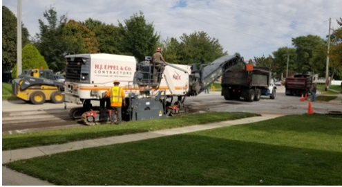
Figure 37: Milling asphalt before resurfacing
