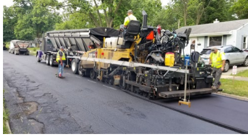
Figure 38: Resurfacing in progress
