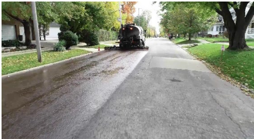
Figure 40: Truck applying Reclamite
