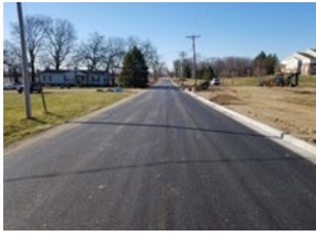
Figure 3: New (10) - New construction. (City) recent overlay. Like new.
