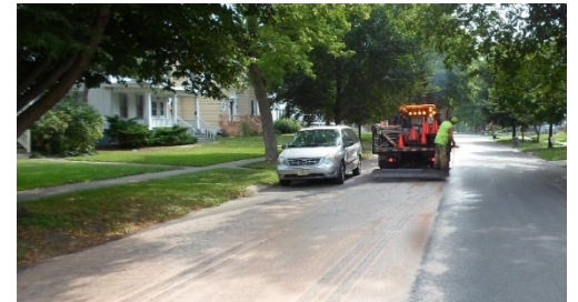
Figure 42: Truck applying sand after Reclamite.
