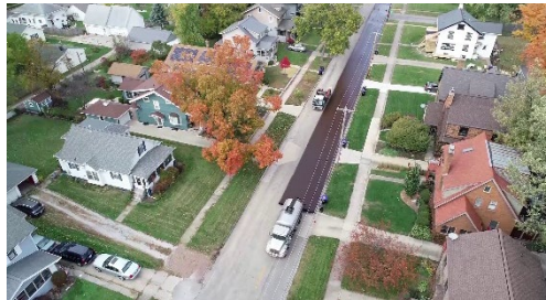
Figure 41: Drone image of trucks applying Reclamite and sand
