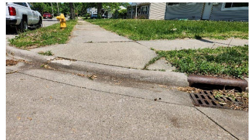
Figure 29: No ramp creates a curb barrier
