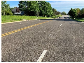
Figure 4: Excellent (9) - Recent overlay. Like new. No cracking.
